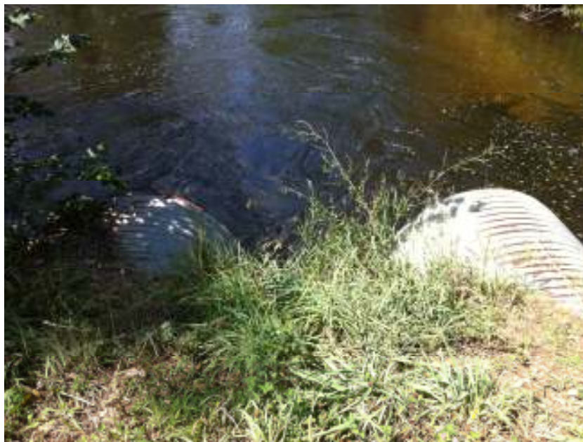
County Drain Culverts
