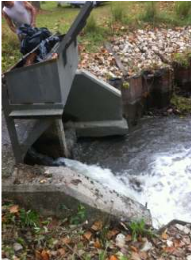
Shavehead Lake Dam
